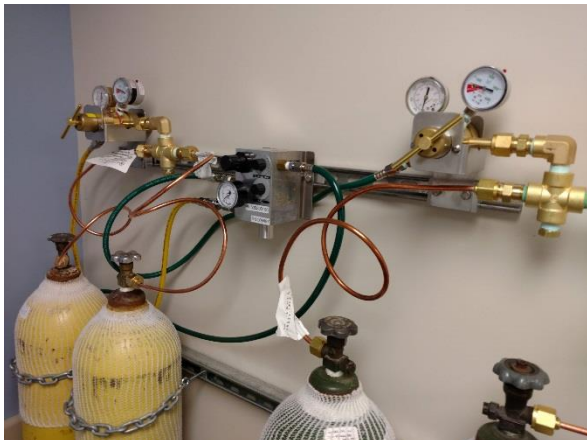
FIGURE 1 MAGELLAN MANIFOLD SYSTEM
